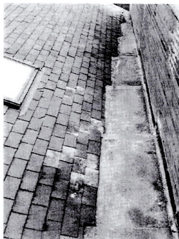
Photo 2 - Broken Slates Replaced
